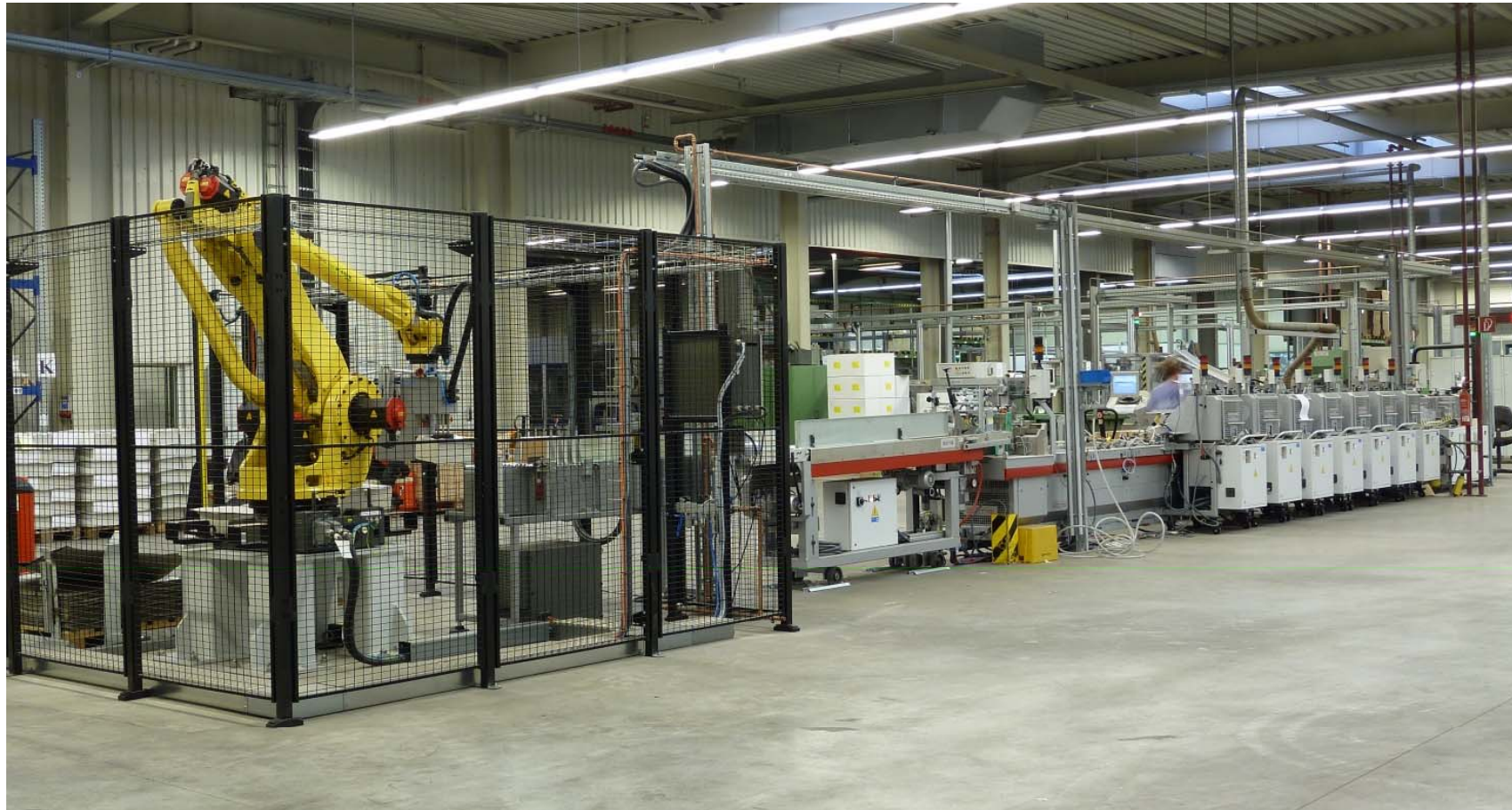
View of the RS 550 Depalletizing Robot and its stack feeder in front of the downstream inserting, film-wrapping, addressing and palletizing line.
